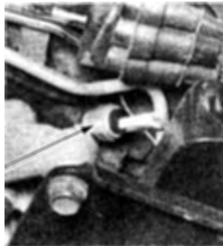
6.1b The coolant temperature sending unit on V6 engines (arrow) is located near the left front corner of the intake manifold
