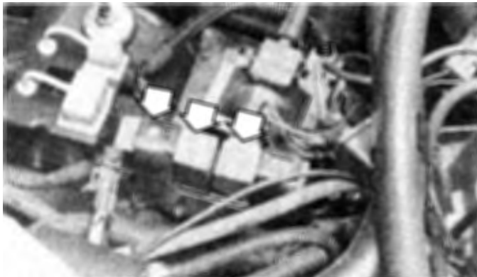
6.2 Three of the relays (arrows) are located in the engine compartment adjacent to the battery, under a cover
