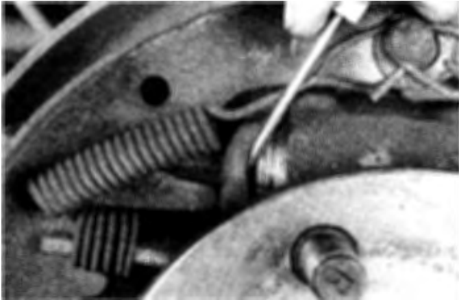
20.14 Peel the wheel cylinder boot back carefully and check for leaking fluid — any leakage indicates the cylinder must be replaced or rebuilt
