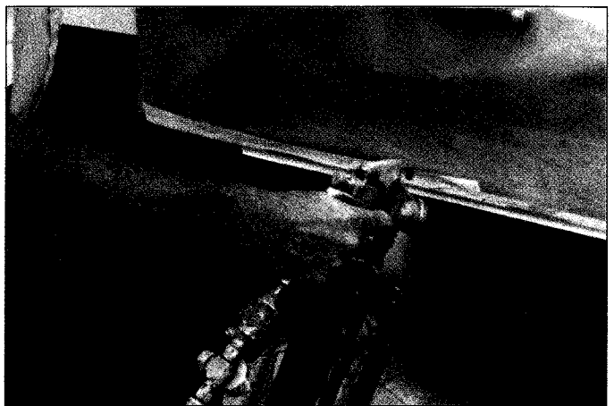
10 Apply several layers of primer to the area. Don't spray the primer on too heavy, so it sags or runs, and make sure each coat is dry before you spray on the next one. A professional-type spray gun is being used here, but aerosol spray primer is available inexpensively from auto parts stores
